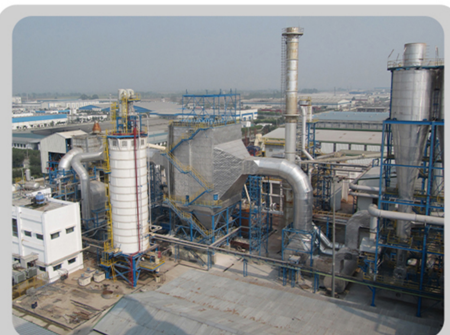
47 MW Energy Plant for an MDF Industry in North India
