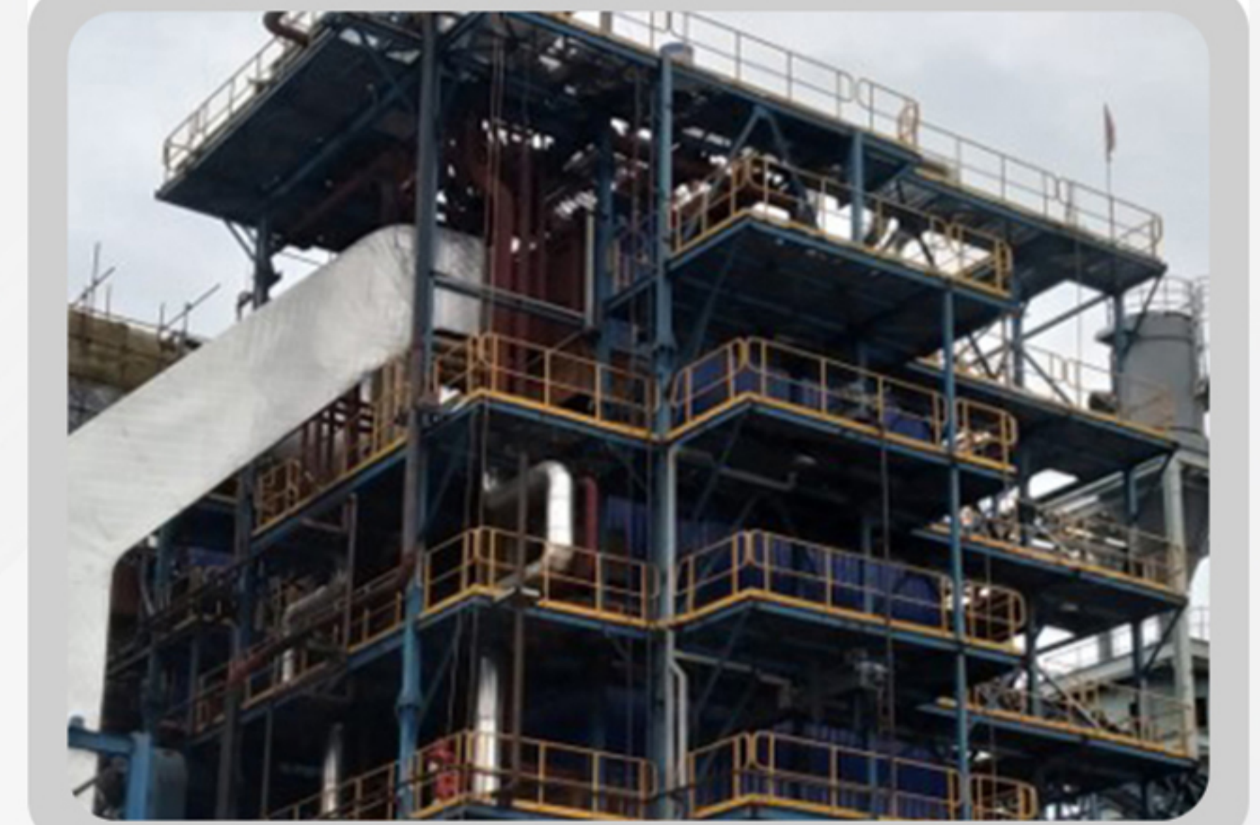
47 MW Energy Plant for an MDF Industry in South India
