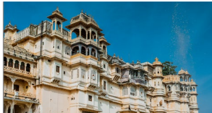
Provided construction chemicals for the restoration of the iconic Udaipur palace in India
