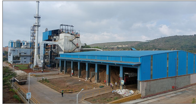
Installed a biomass-based cogen plant for an aluminum major in Karnataka, India
