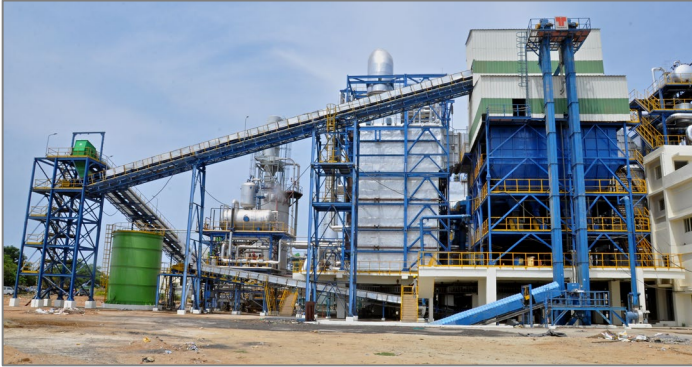
An energy plant of 97 MW commissioned for a plywood major in Andhra Pradesh, India
