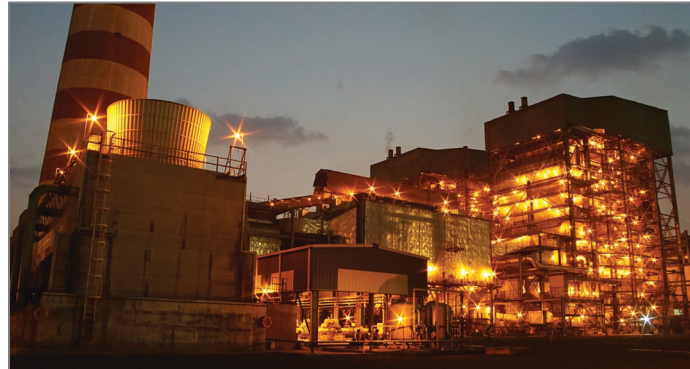
A 300 MW independent power plant set up for a power generation company in Telangana, India
