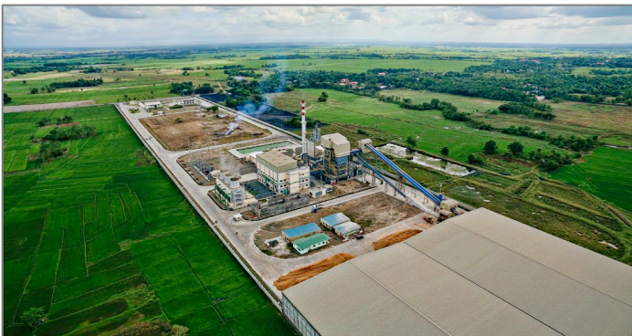
100% rice husk fired independent power plant set up for an energy corporation in Philippines
