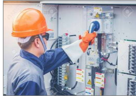
O&M for a 90 MW captive power plant for an alumina refinery in Odisha, India
