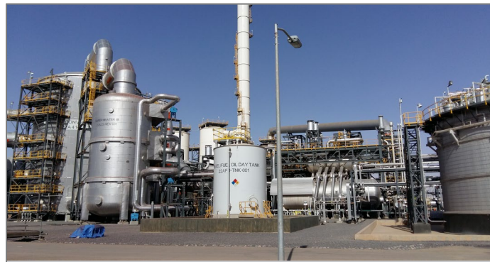
Supplied 3 X 261 TPH waste heat recovery equipment for the largest phosphate plant in the world at Saudia Arabia
