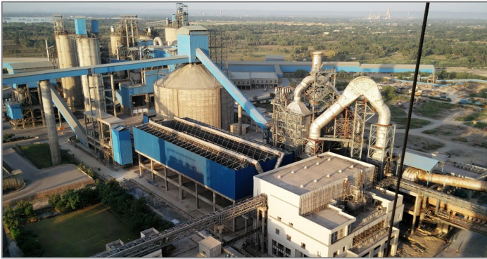
An 18 MW waste heat recovery power plant set up for a cement major in Rajasthan, India
