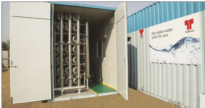
Installed a water treatment plant at a fertiliser MNC located in Jordan
