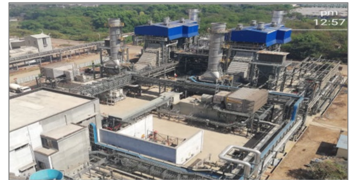
A 50 MW gas based cogeneration plant set up for a chemical major in Maharashtra, India
