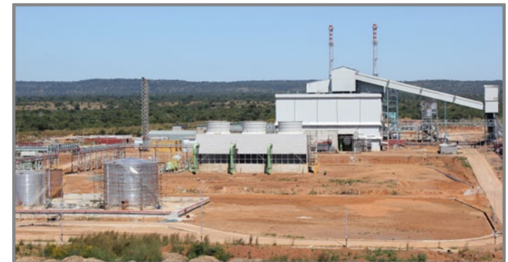
A 30 MW captive power plant installed for a cement company of a major conglomerate in Africa
