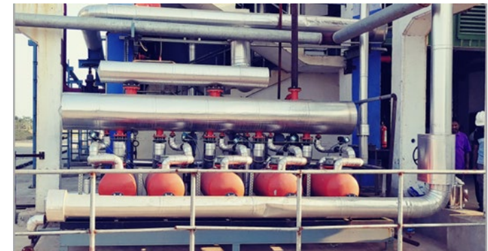
55 TPH condensate recovery pump (five plex) successfully installed for a leading pharma company in Andhra Pradesh, India
